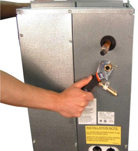
Slowly loosen nut on suction line. Coil is pressurized with nitrogen which will be released.
