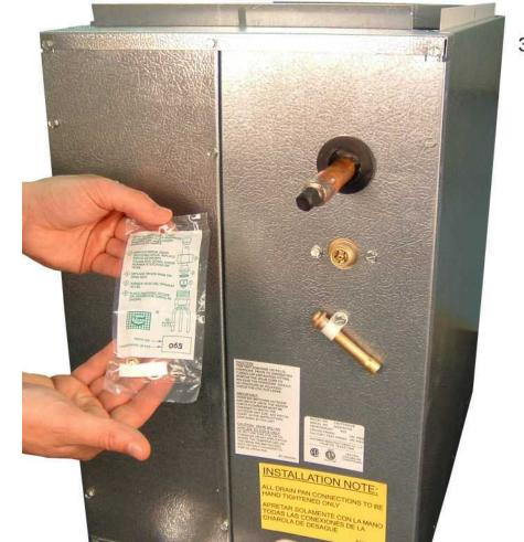
3. Locate replacement orifice kit which is provided with most Goodman condensing units.
