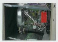
Lennox's control board must be removed in order to remove the blower
