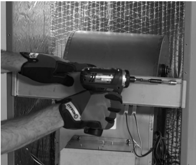
Installing Support Bar
