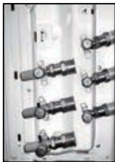
Tighten quick connectors
