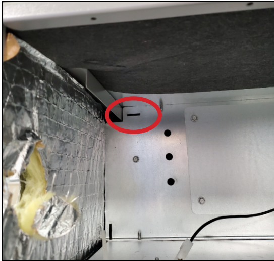
Figure 12. Notch for Control Panel Relocation
