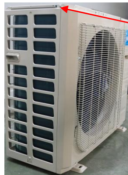
Screws of front panel
