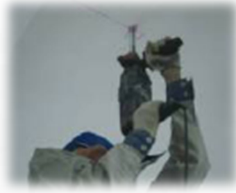
Drill holes on the ceiling
