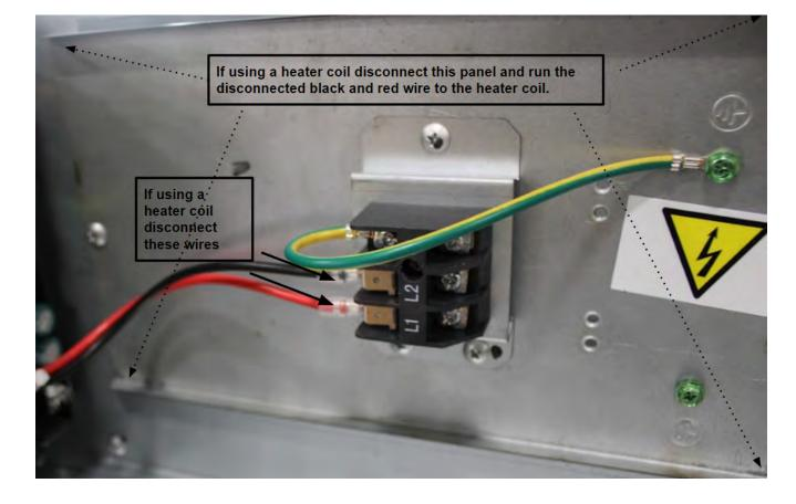
If using a heater coil disconnect the red and black wires above, and cut back any attached connector and strip 1/2 of insulation from the end of the wires. Then remove the panel and run the disconnected black and red wires to the heater coil. Follow the instructions below to supply the air handler with power when installing a heater coil in the BMAH series of air handlers.
