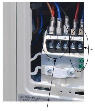
L1 L2 are the incoming power. Either hot wire can connect to either L1 or L2 ground goes to any green ground screw.
