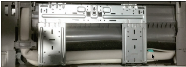
Line set connection cap. Loosen to check for pressure. You should hear a hissing sound
