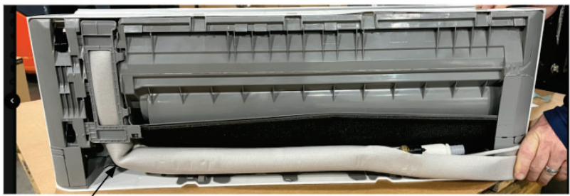
Line set connection pivot point
