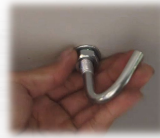
Insert the expanding hook into the hole and hang in the suspending rod.
