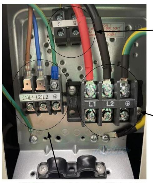
(1)L1 (2)L2 and ground . Connect the 14/4 wires to these terminals and match the same wire color with the same terminal on both the indoor and outdoor unit. You will not use the 4th wire. We recommend Black on (1)L1 Red on (2)L2 and green for ground
